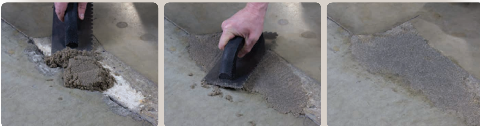
Apply mix to damaged area and smooth with trowel
