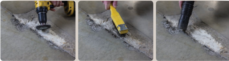
Prepare damaged area
