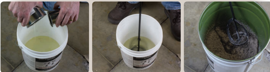
Mix liquid parts A & B, then slowly add sand
